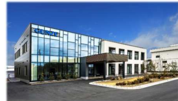
New ZEB office building in Konan
