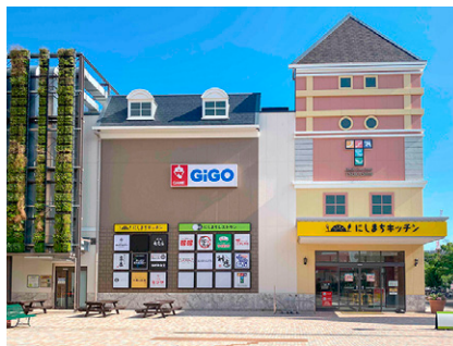
Exterior of Nishimachi Kitchen at Gunze Town Center Tsukashin
