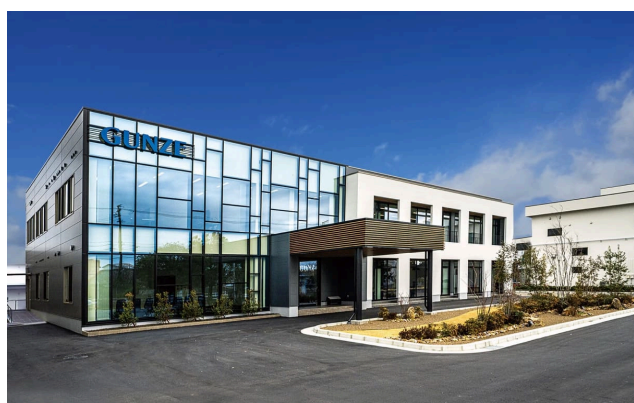
The Konan Plant's ZEB office building
