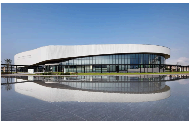
Exterior of the Kurunto facility
